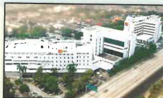
Sime Darby Medical Centre, Subang Jaya
