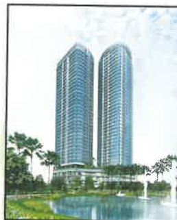
UOA Vertical Hotel, Bangsar South
