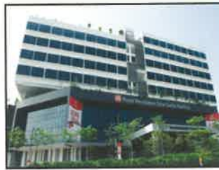
Desa Park Hospital
